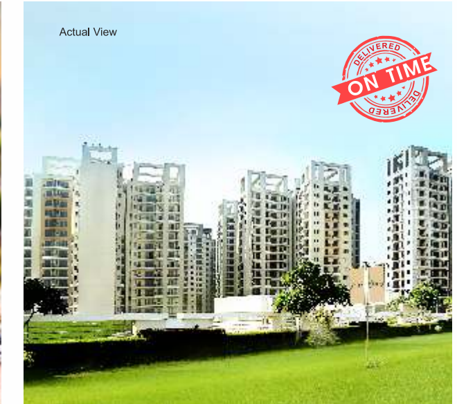
Phase - I: Completion Year: 2017 Covered Space: 940065 Sq Ft Approx Total No Of Units: 756 RERA REGN. NO: RAJ/P/2017/075
